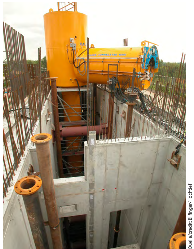
Flughafen-S-Bahn Hamburg, Caisson Baulos 7 Airport Light Rail Hamburg, Caisson Lot 7
