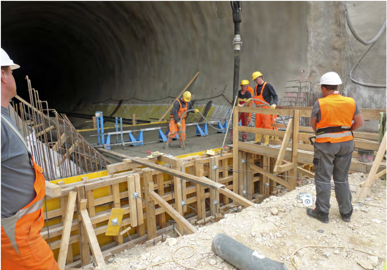
5 Betonage erster Sohlblock, Steinbühl Tunnel Süd, Oströhre Concreting of the first invert block, Steinbühl Tunnel South, east bore
