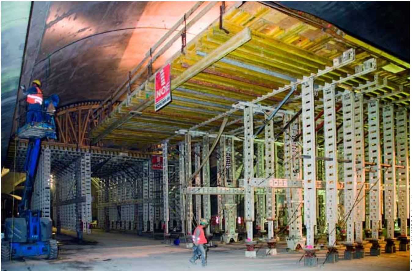
NOEtec formwork carriages for the emergency bay (left) and ventilation gallery (right) NOEtec Schalwagen für Pannenbucht (links) und Lüfterstollen (rechts)
