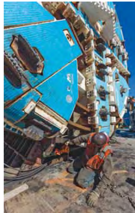
Montage des Bohrkopfes Installation of the cutterhead
