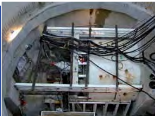
Shaft installation, Wientalsammler, Austria
