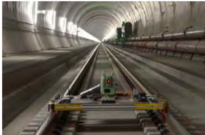
Messwagen zur Kontrolle der Gleislage Measuring car for checking the track position
