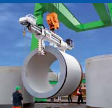
Crossbar for lifting concrete pipe segments
