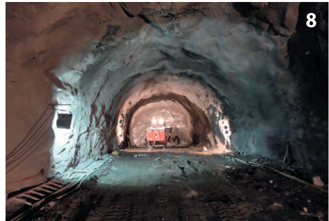
After the shotcrete, technicians inspect the surface of the area to continue the drilling works.
