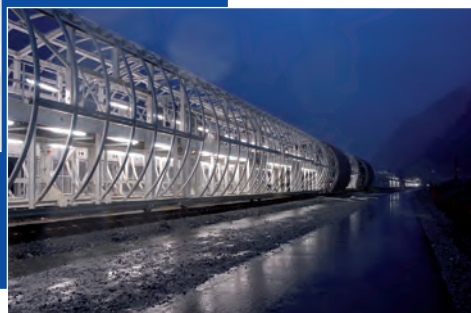
Back-up system „Worm“, Gotthard Base Tunnel, Switzerland
