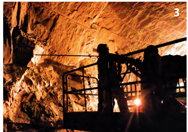
Installing support bolts
