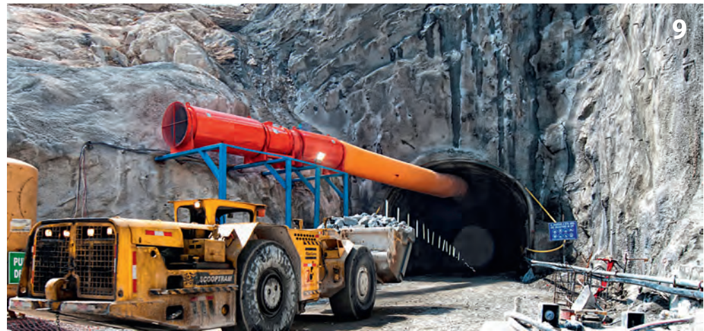
Portal of the Punta Olimpica Tunnel with the ventilation system being installed
