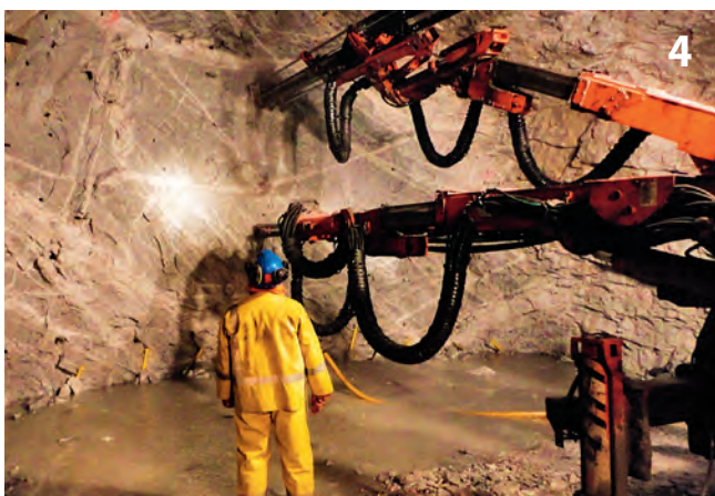
Tamrock jumbo with its massive arms in operation
