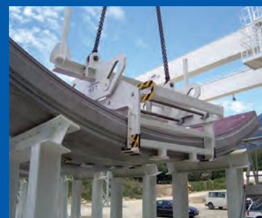
Segment handling system Mont Sion, France
