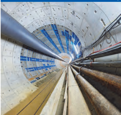
Steel tunnel segments, Wehrhahn Line Düsseldorf, Germany
