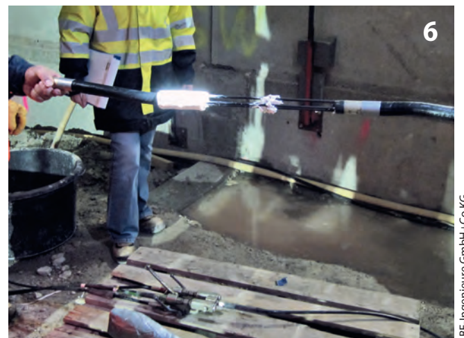
Detail der Probeinjektion Detail of the trial injection
