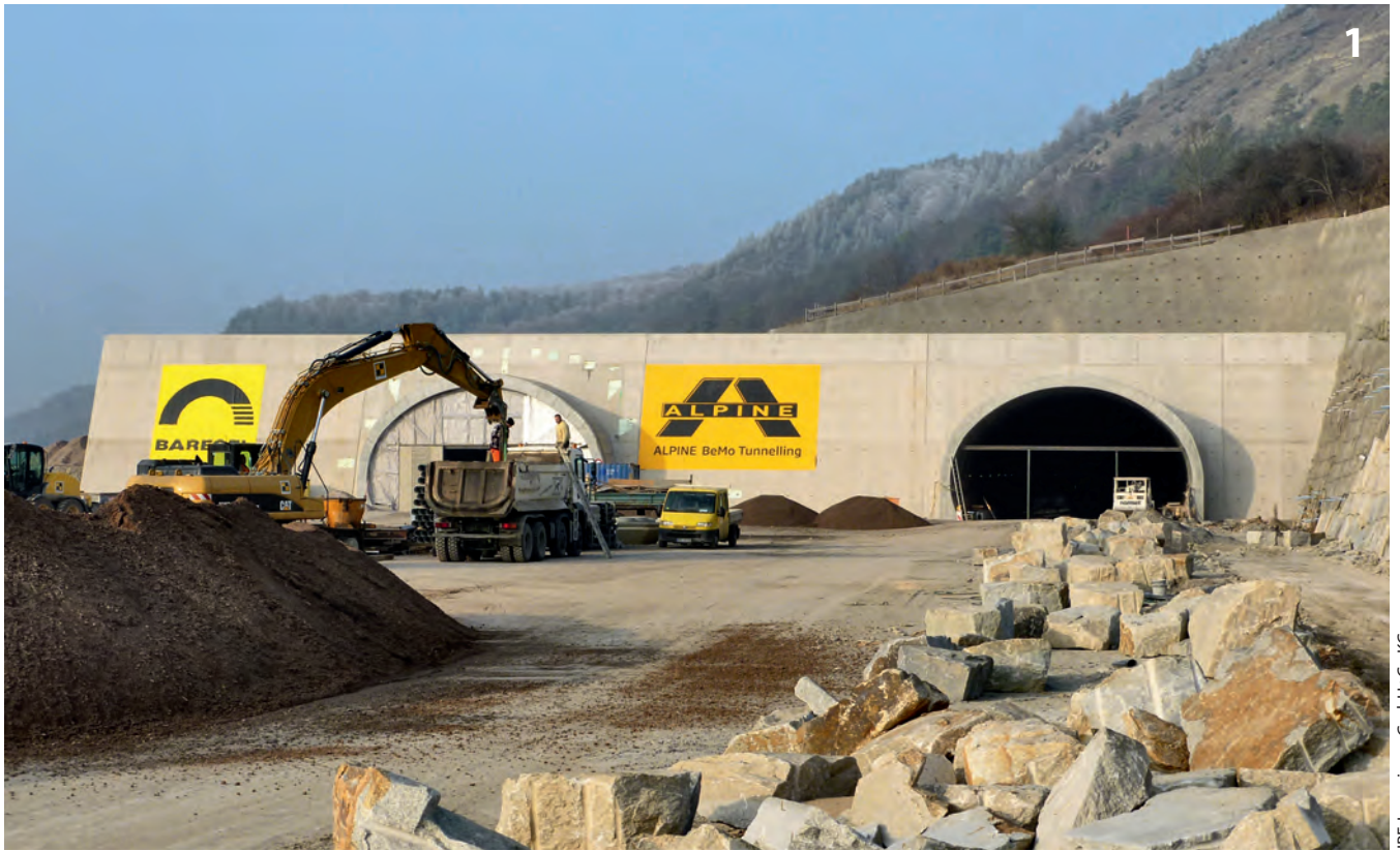
Ostportale des Jagdbergtunnels East portal of the Jagdberg Tunnel
