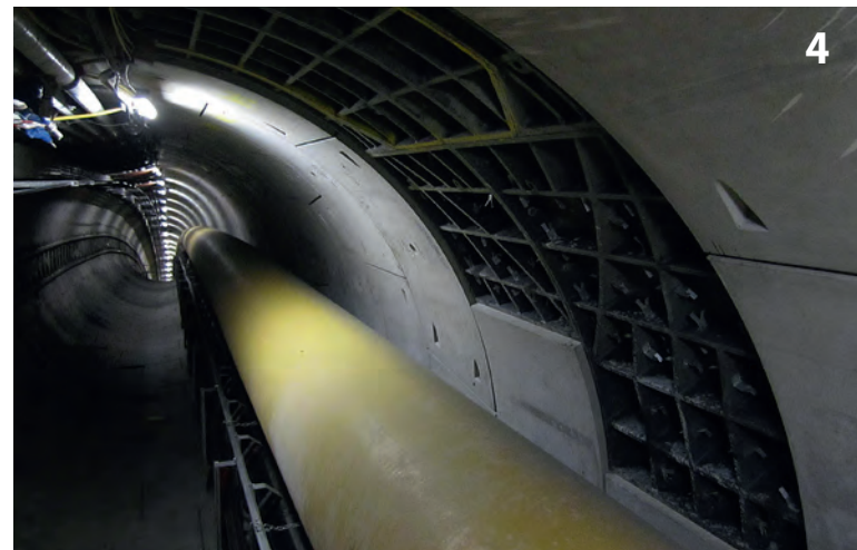
Tunnelschale Westbound Tunnel mit SGI-Öffnungs-Set CP01 Westbound tunnel shell with SGI opening set CP01
