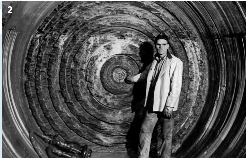
James S. Robbins stands in front of an early TBM excavation face showing kerf cutting
