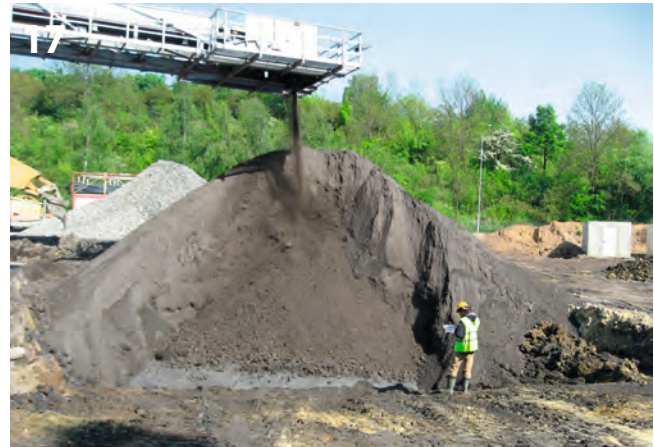
An initially good result of the "dry" muck production attempt, which failed after 75 m with the ingress of the groundwater and generation of sticky muck
