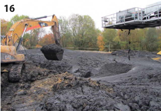
The clayshale rock was transformed into a mud by large quantities of water added to the cutterhead
