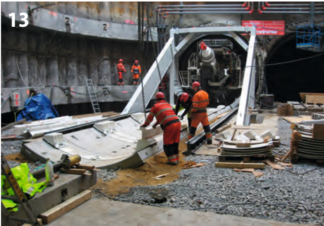
Massive bracing frame for EPBM start in the circular launch shaft
