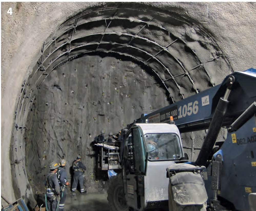
Execution of services in the region of the Soriman fault
