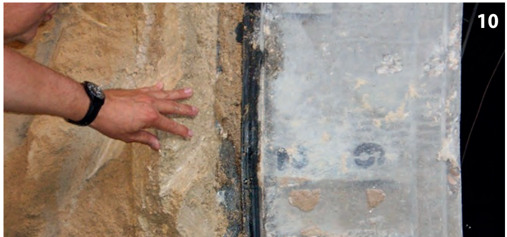
Verpresster Ringspalt Grouted annular gap
