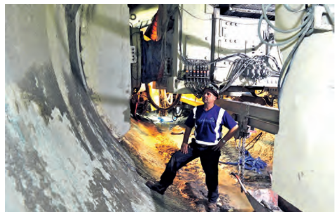
Adit 4 Site Manager Andy Birch (Robbins) surveys the excavated tunnel
