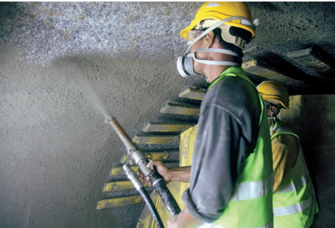
A novel type of polypropylene fiber shotcrete is being applied as the primary means of ground support - a mixture that reduces rebound
