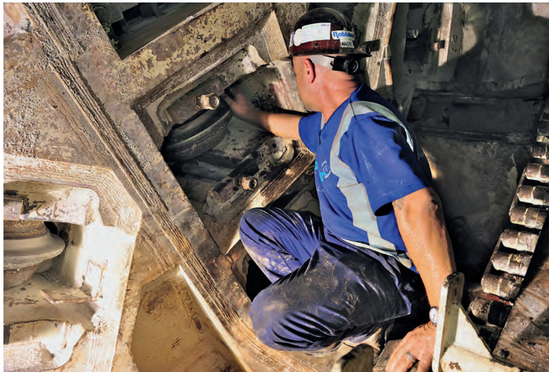
The remote cutter monitoring system, which enables continuous tracking of cutter wear, has been installed on 1 of the 3 TBMs
