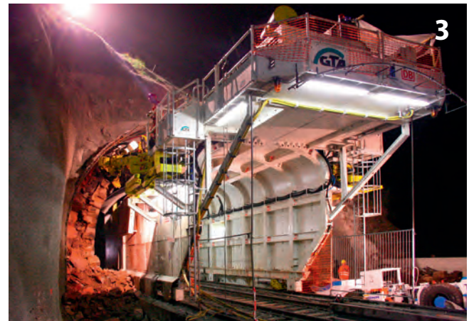
Tunnel-im-Tunnel Vortriebsportal Tunnel-in-tunnel driving portal
