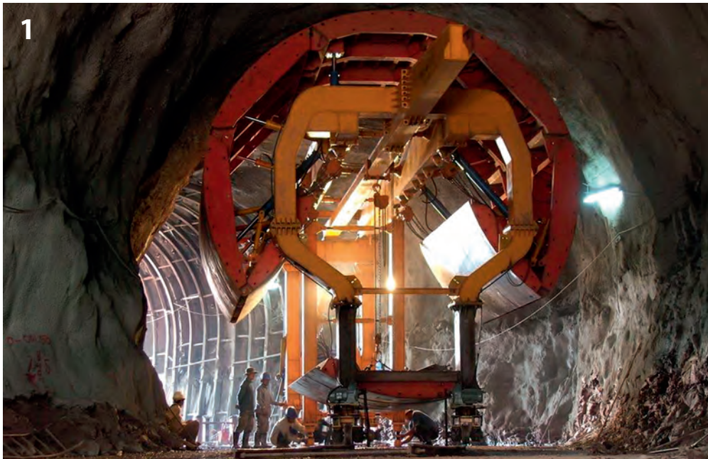
In Thailand are various tunnels under construction
